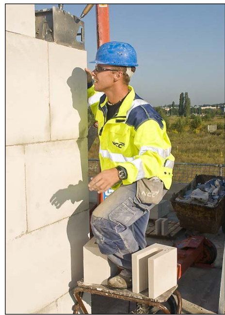
Figure 6 The German platform: achieving value creation and cost reduction by using 60x60 cm modules
