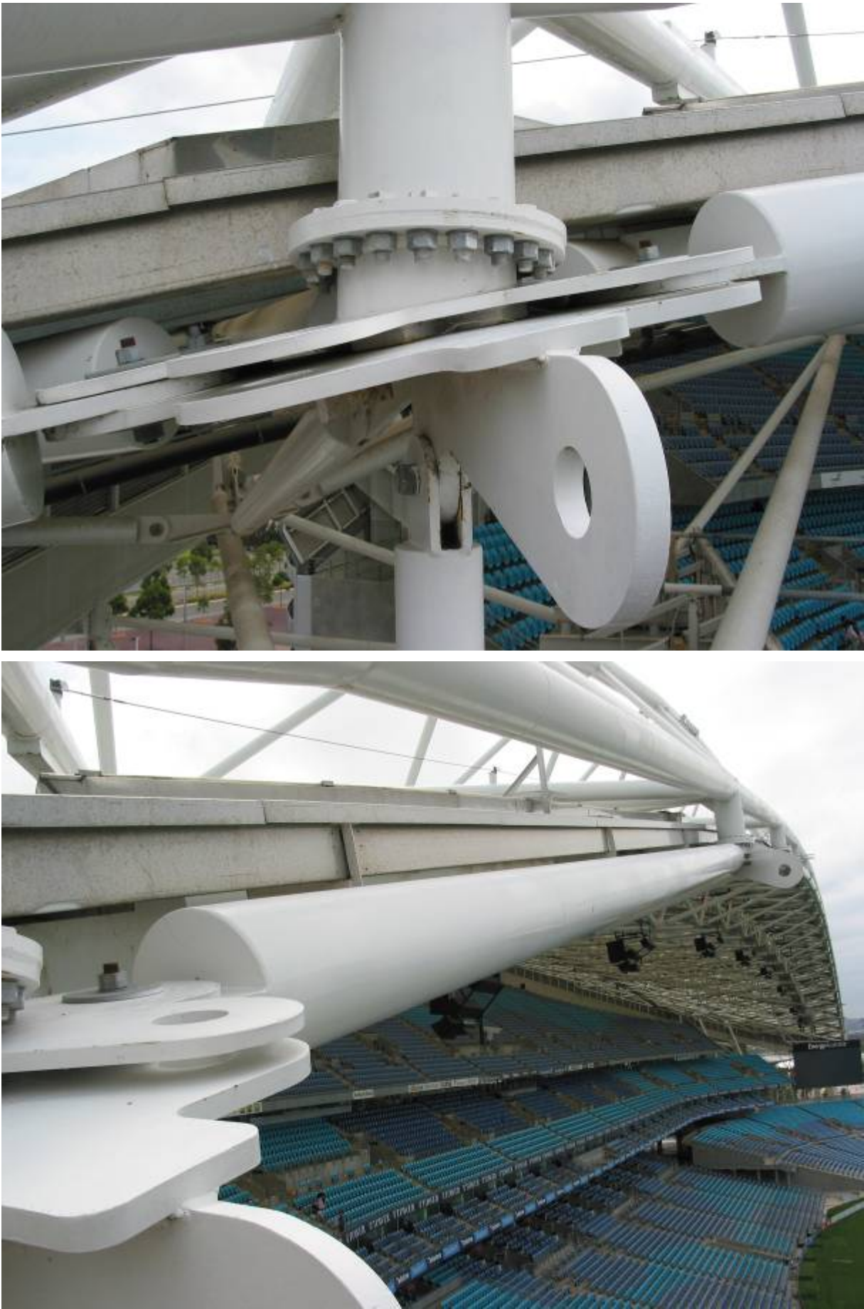
Figure 5 Bolted intermediate sections
