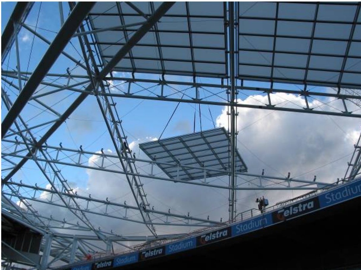
Figure 6 Lifting and installation of the poly-carbonate roof panels
