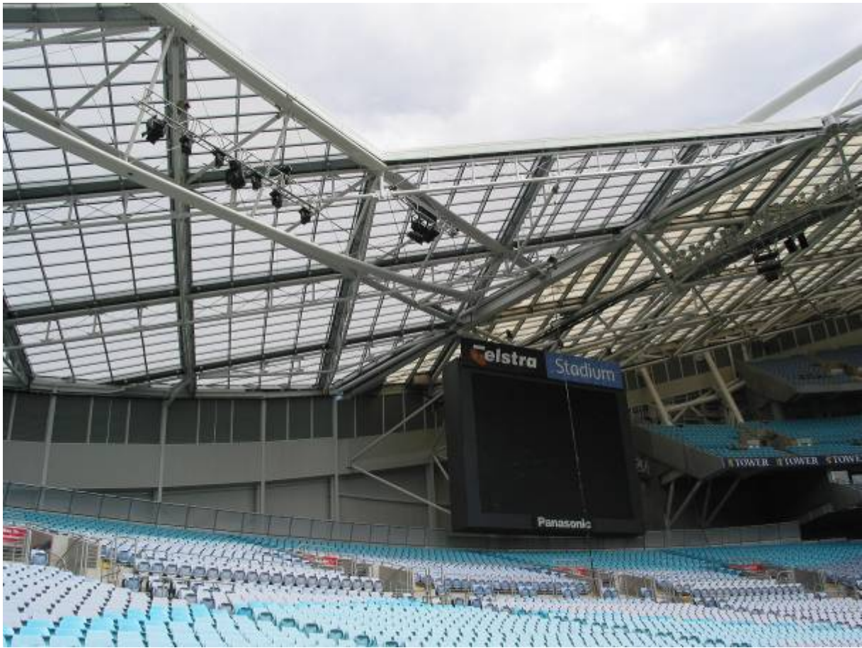
Figure 2 Newly built undercover seating in Stadium Australia
