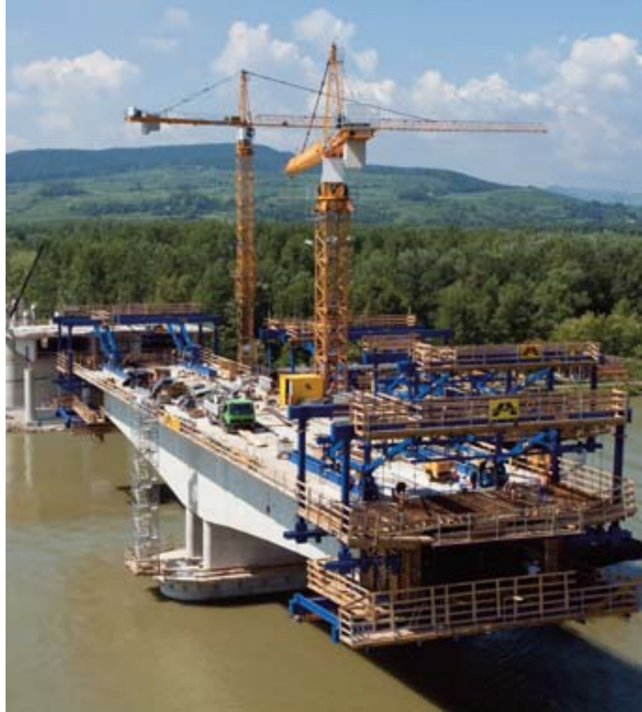
Construction of Traismauer Bridge over the Danube (Lower Austria).
