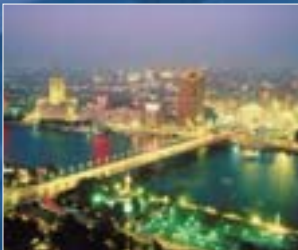
FCC to build waste water treatment plant in Cairo, Egypt. Page 36
