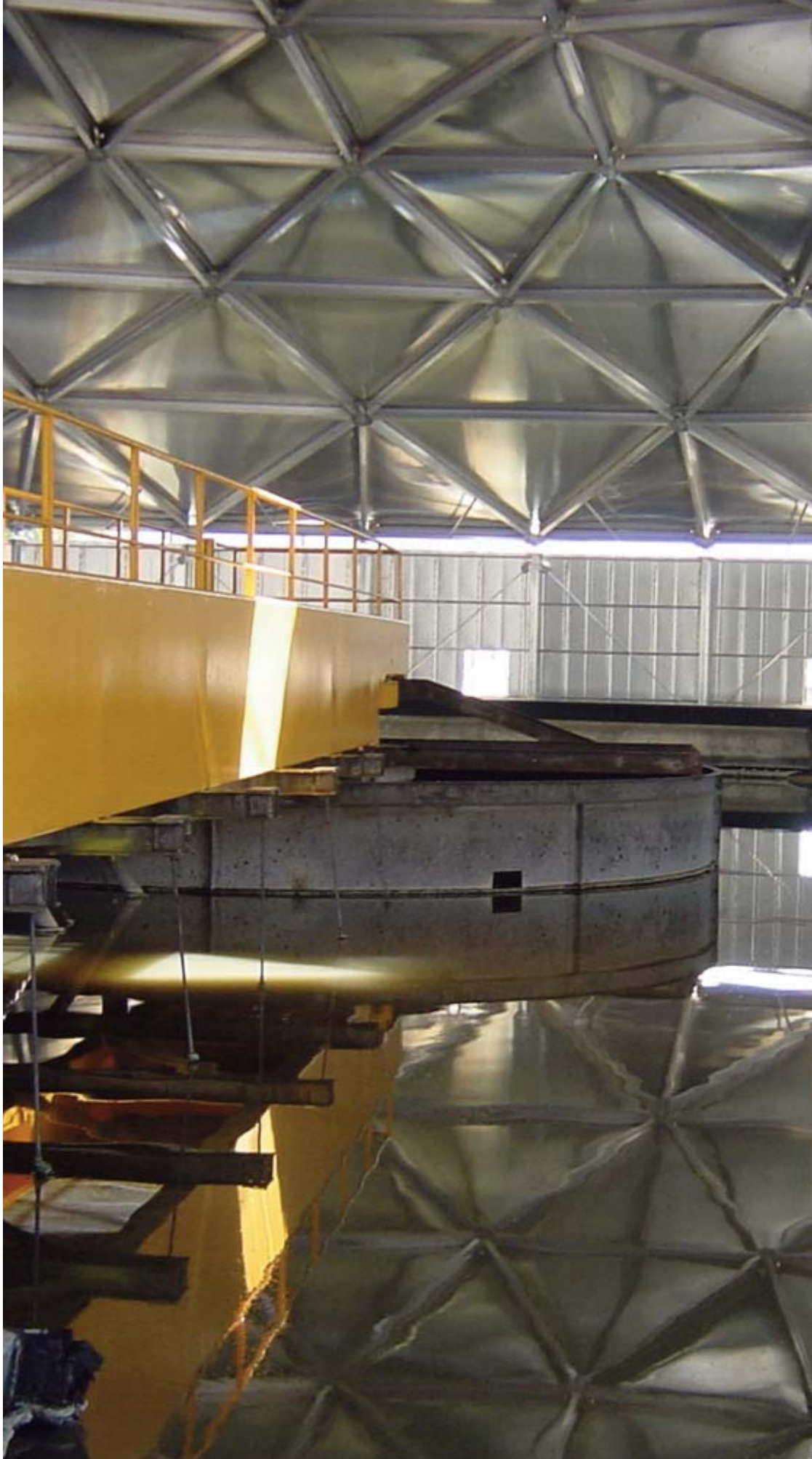
The FCC-built Casaquemada wastewater treatment plant in San Fernando de Henares, Madrid.
