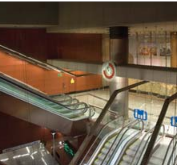
The Puerta del Sol station consists of two main parts: the cavern housing the platforms and the vestibule which provides access to the station and connects with the subway system.
